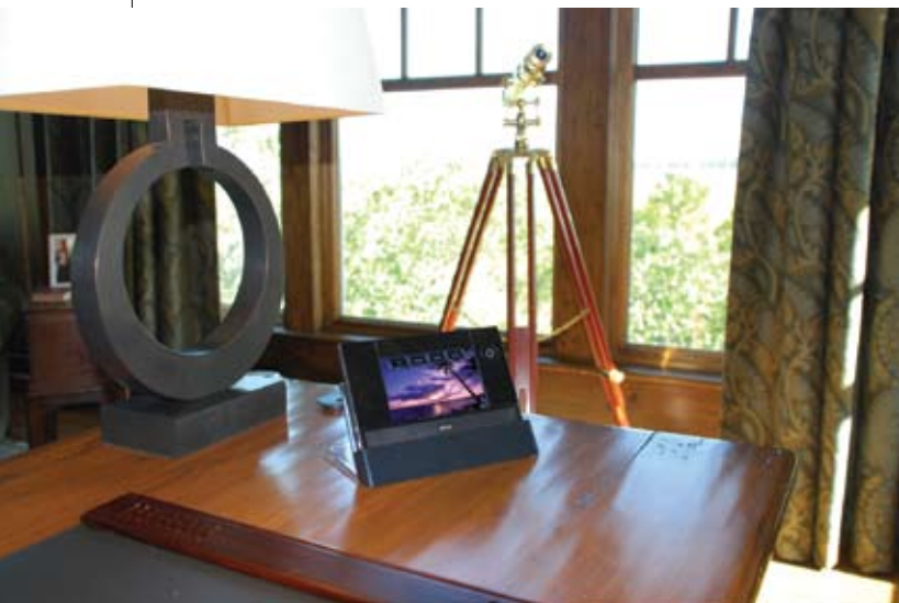
The study in a Kiawah Island home equipped with the Home Cyber Shield monitors 46 IP-addressable devices, including an AMX control system.
